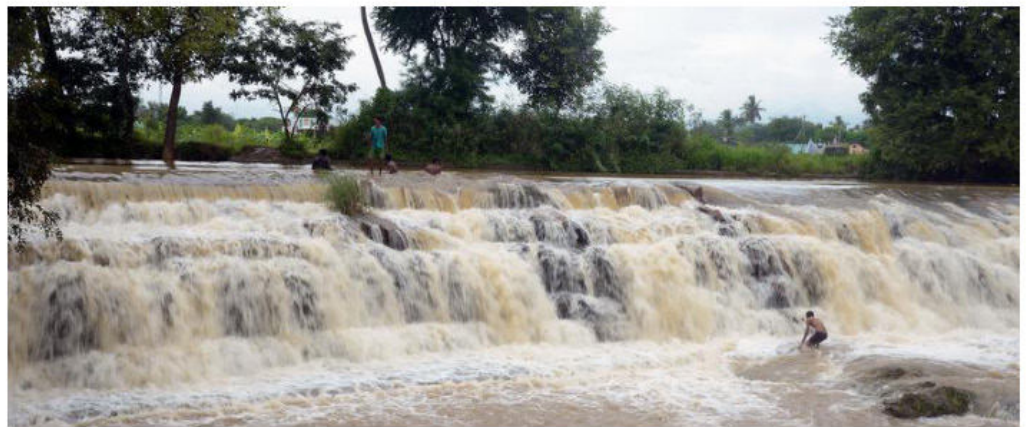
In full flow: The check dam on the Kudaganar river near Dindigul witnessed heavy flow on Wednesday thanks to the recent rain. G. KARTHIKEYAN
